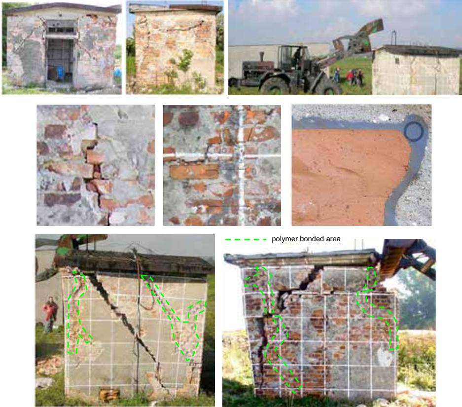
Figure 4. Seriously cracked masonry building repaired by injected PUFJ and efficiently protected against dynamic loading caused by a caterpillar [6].
