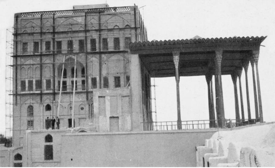
Figure 4. Ali Qapu building, using horizontal circumferential frame in the whole building in order to prevent the external parts from detaching, 1964-1970 (after Galdieri [5]).
