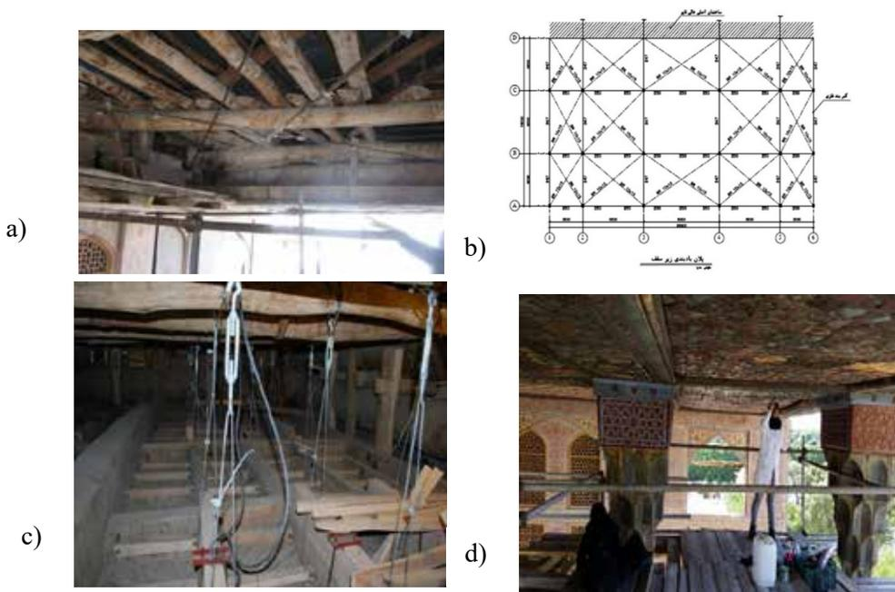
Figure 12. Ali Qapu building, the roof of the wooden columnar structure: a) and b) adding steel cables as the lateral load bearing system, c) and d) supporting the hanging ceiling by steel hangers (2005 to 2017).
