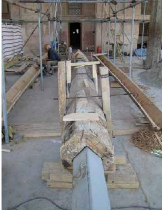
Figure 9. Ali Qapu building, stiffening wooden columns with steel profiles (2005 to 2017).
