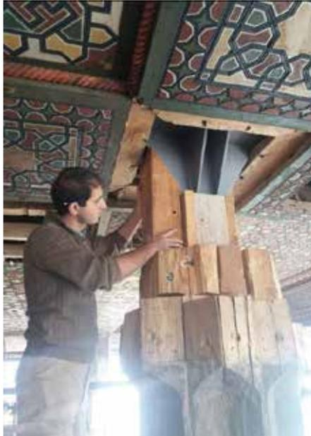
Figure 11. Ali Qapu building, strengthening the connections of the columns to top beams (2005 to 2017).
