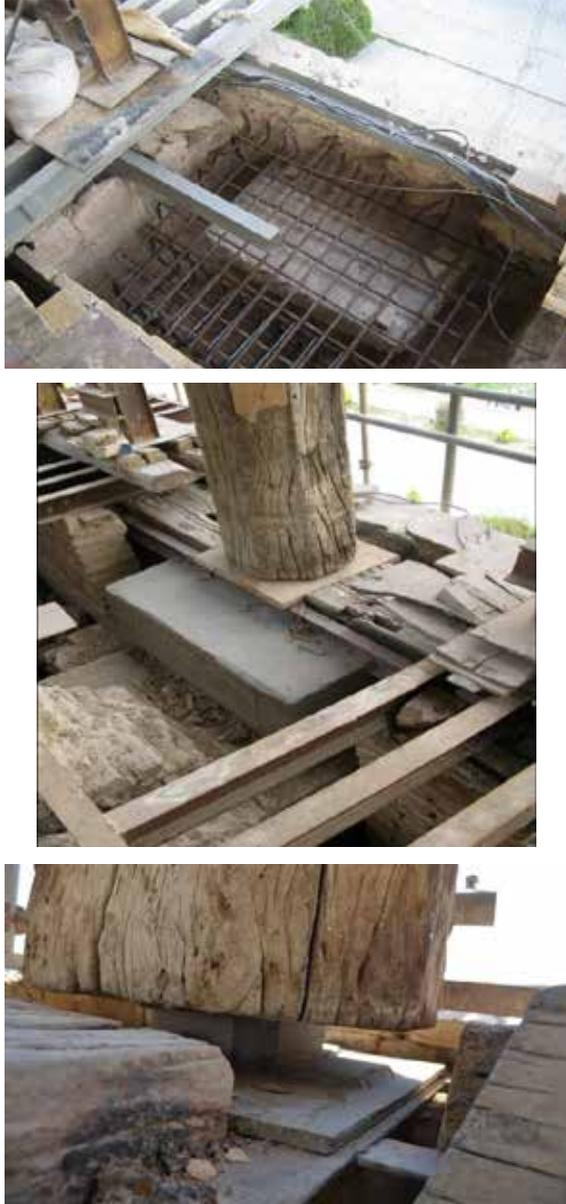
Figure 10. Ali Qapu building, strengthening the supports of the columns (2005 to 2017).
