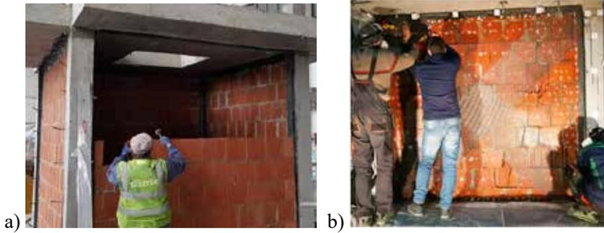
Figure 3. Installation of: injected and prefabricated PUFJ (a), FRPU composite (b).
