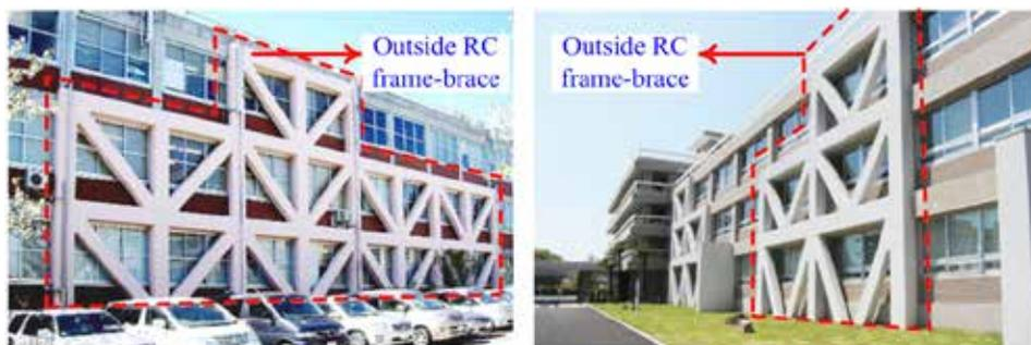
Figure 1. External retrofitting by RC braced frames (Cao et al., 2020)
