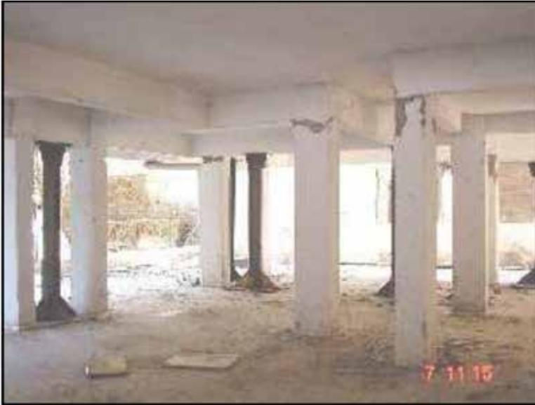
Figure 3. Columns damaged by the effect of discontinuous beams [1]
