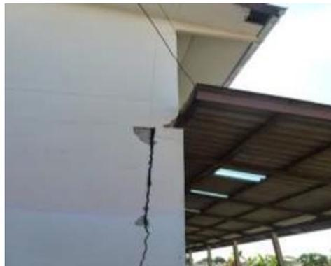
Figure 1. School buildings : Observed damage on buildings in Thailand by Mae Lao earthquake
