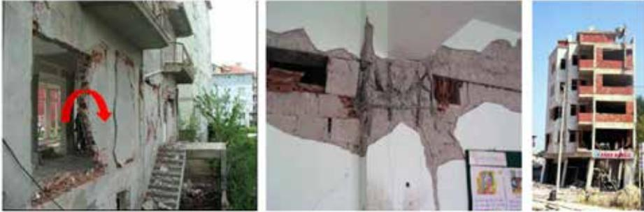
Figure 1. Infill wall related failures after earthquakes; in-plane and out-of-plane damages (left) [3], corner crushing of the wall and shear damage on column (middle) [4], and soft-story mechanism (right) [5].
