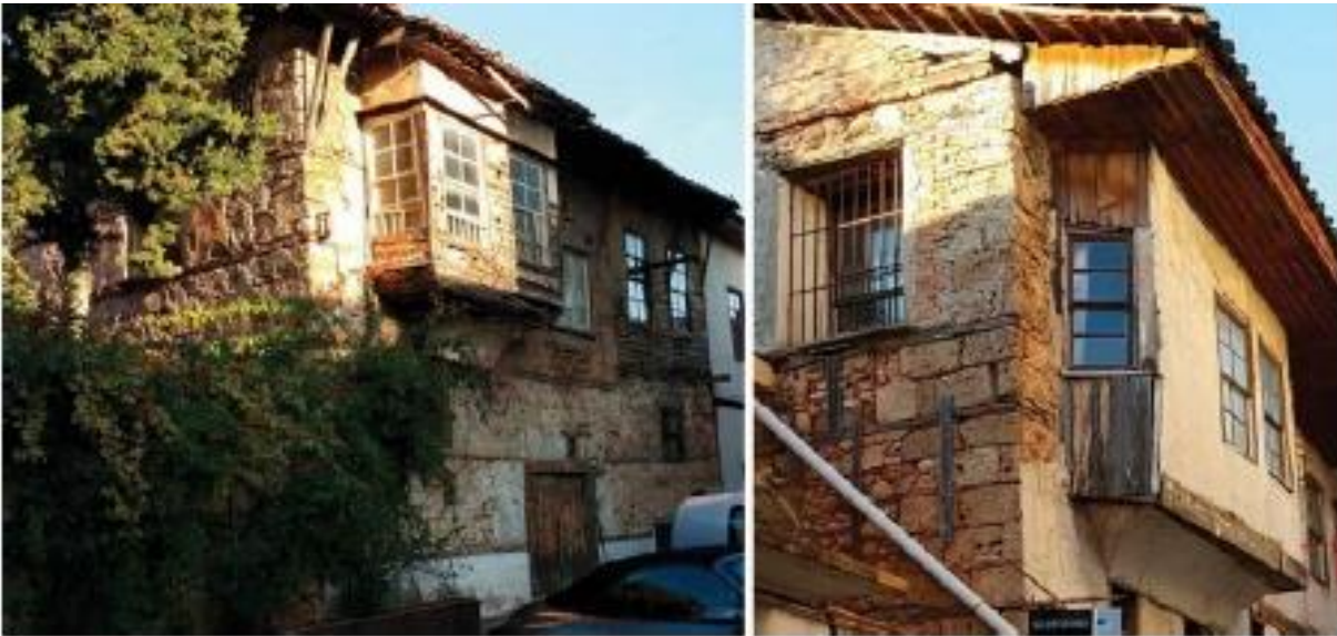
Figure 6. Right: Stone used as a cornerstone (pillow stone) in the corners of the wall (Author). Left: Construction system of the houses' ground and upper floors (Author)
