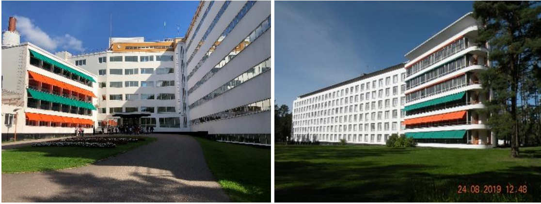
Paimio Sanatorium main entrance, patient care ward and sunning terraces (photographed by author, 2019)
