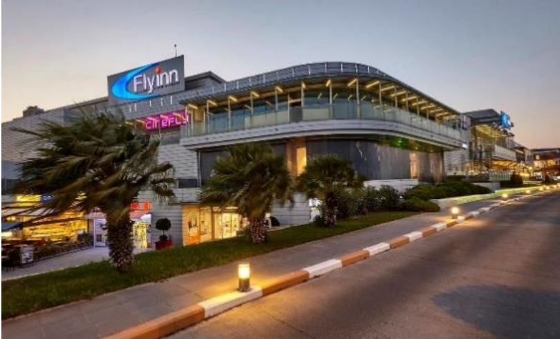
Figure 2. Flyinn Shopping Center Front Facade View [14].
