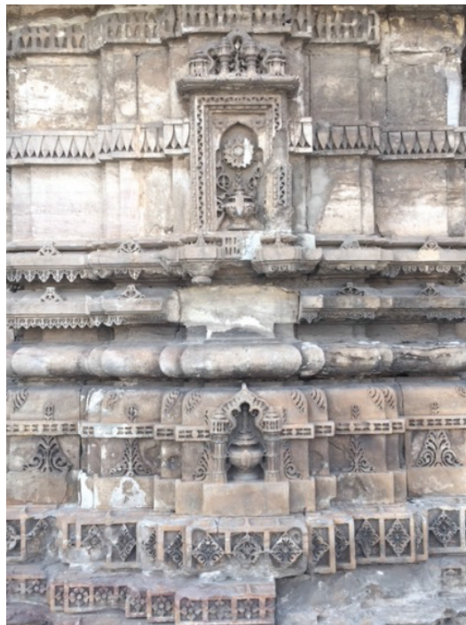
Figure 2. Elements of Hindu Architecture at Jami Masjid
