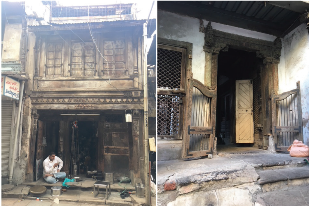
Figure 4 and 5: Typical facades of pol houses
