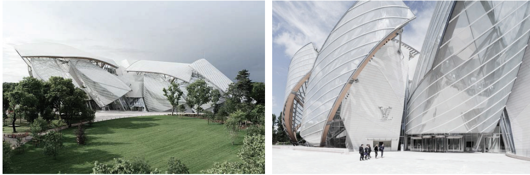
Figure 4. Foundation Louis Vuitton, Frank Gehry, Paris, France, 2014 [20]
