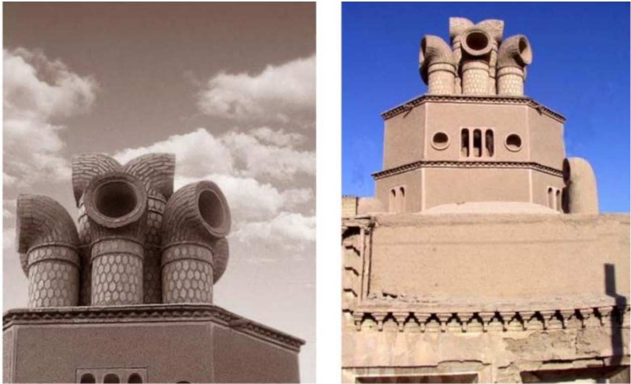
Figure 10. View of wind catcher type 6: pipe like (Chopoghi) [9]
