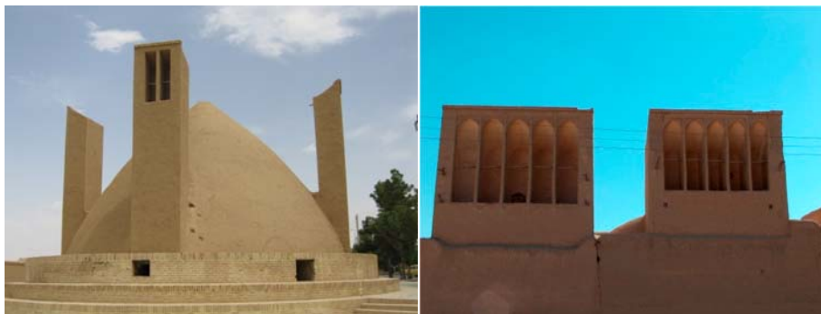
Figure 3. View of wind catcher type 1: one sided; right picture: A view of a one-sided wind tower in Ardakan city, Yazd province, Iran [7]
