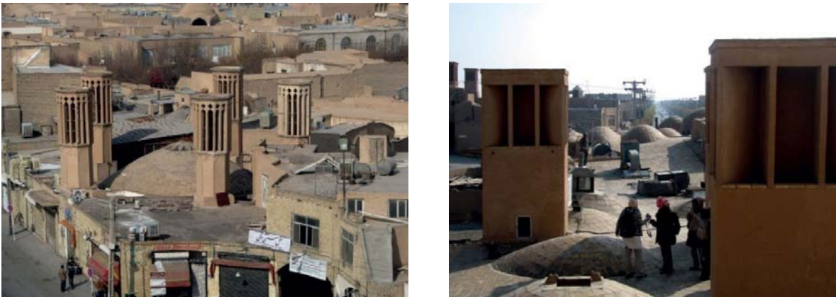
Figure 2. Traditional wind catchers in the city of Yazd in Iran [3]
