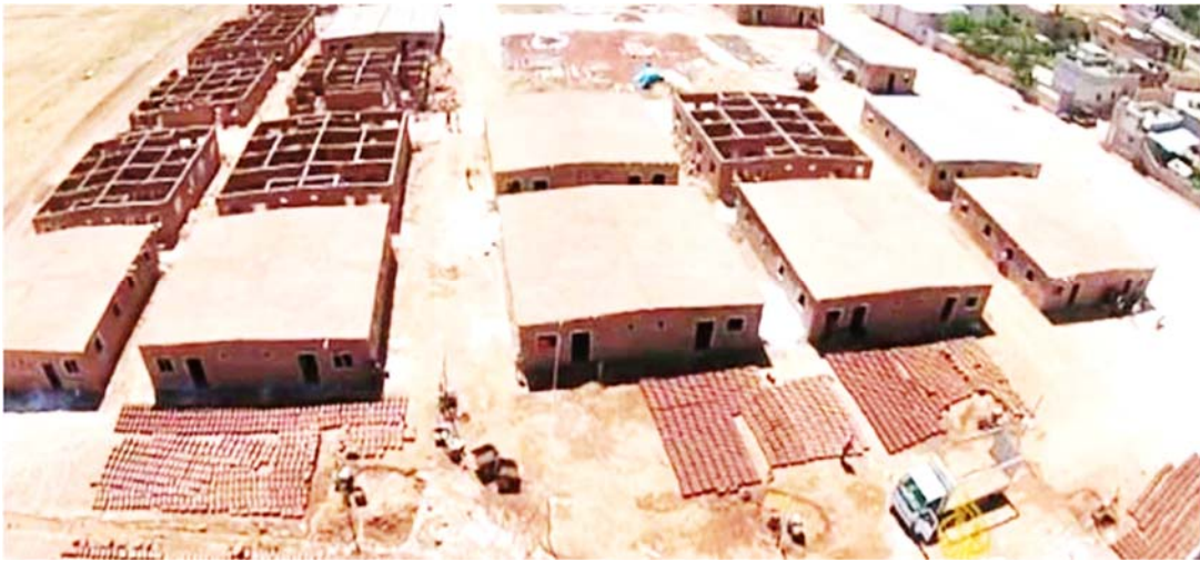
Figure 3. Earthen buildings, Syria [14]
