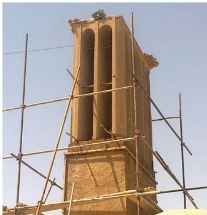
Figure 5. View and dimension of wind catcher type 2: two sided [10]
