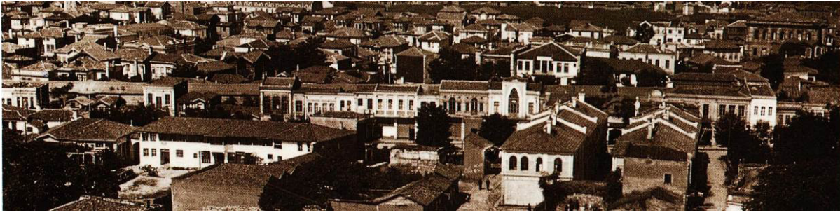
Figure 4. The general appearance of Saraçlar Street in the early twentieth century.
