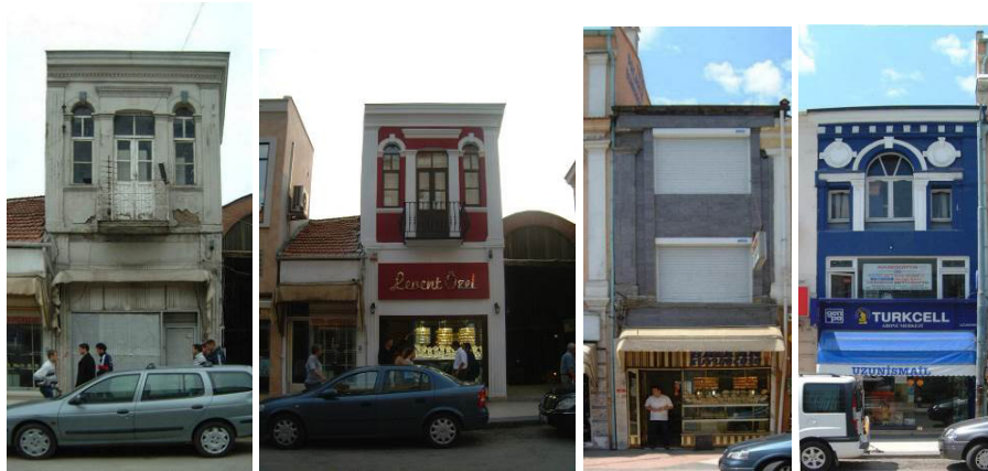
Figure 7. Façade changes along Saraçlar Street.
