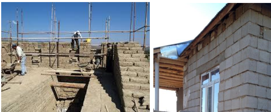
Figure 5. The construction of adobe wall
