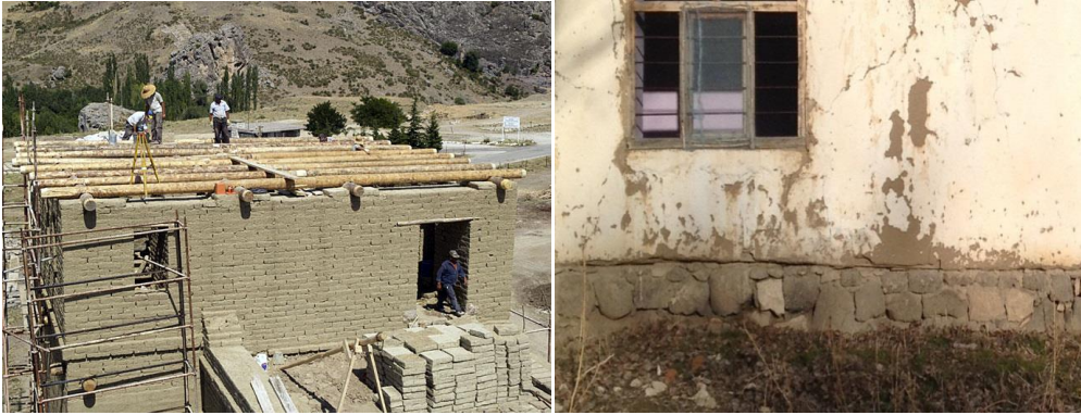
Figure 3. Village of Karahan / Van / Application of wooden roof [4]
